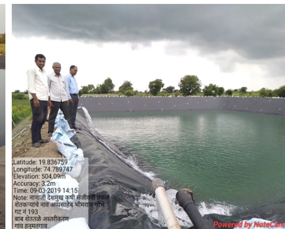
Lining of Farm Pond, Hanumant Gaon, Aurangabad
