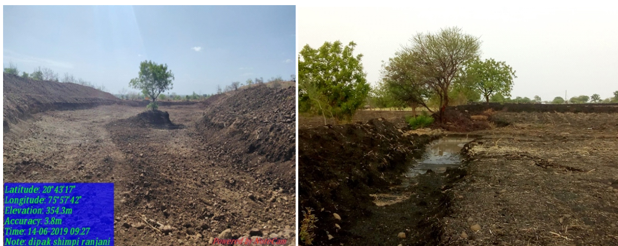
Deepening Of Nala, Ranjni, Tal- Jamner Compartment Bunding, Shelgi, Dist. Latur
