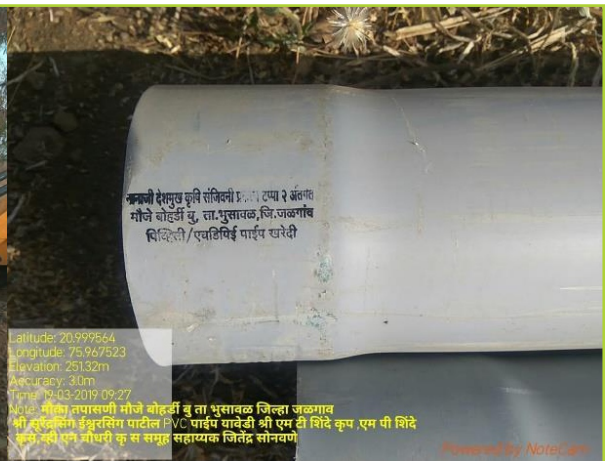
Marking on Pipes Bohardi, (Bk) Tal. Bhusaval, Dist. Jalgaon
